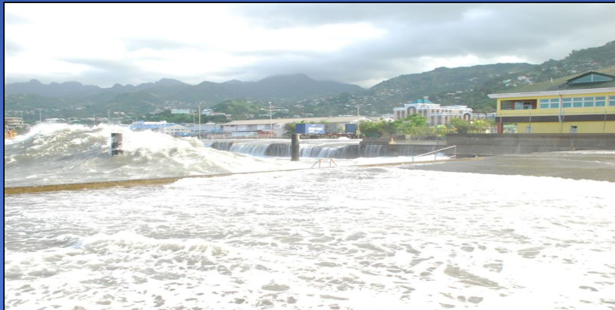
Fig. 9. Storm surge at Cruise Ship Berth- Kingstown
